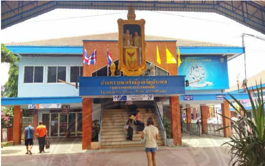
Check point building Thailand side
