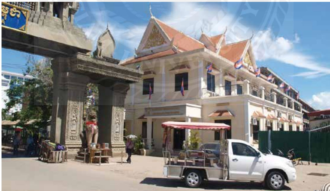
Check piont building Cambodia side under constrution 2018
