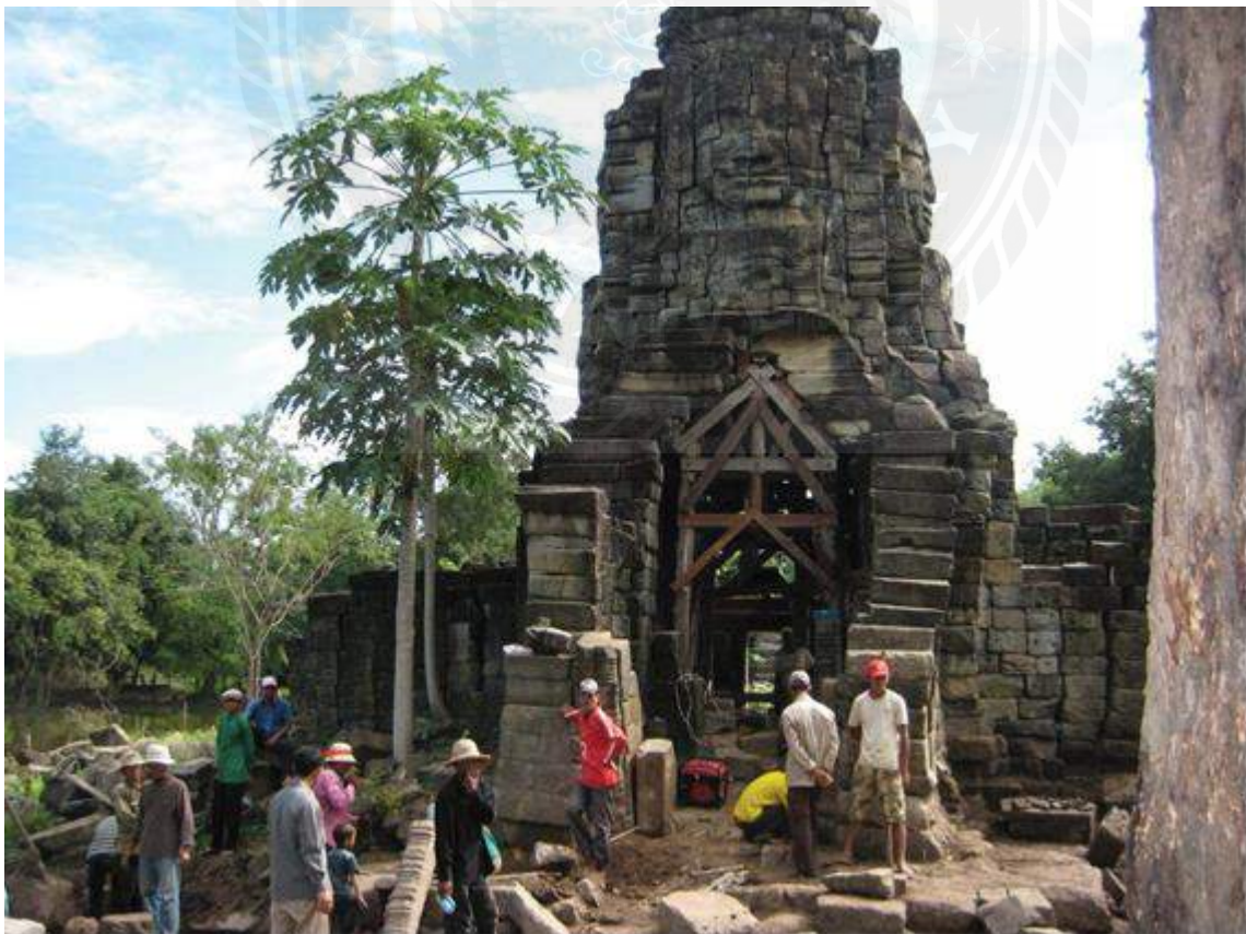
Image 5 Ta Prohm temple (under restoration) (Source: Sotear Ellis)
