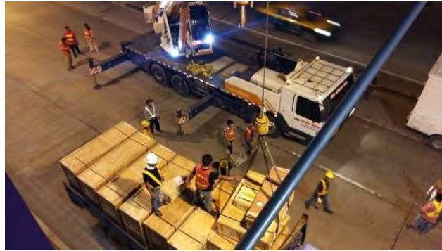
Figure 5-1 AG Hardware Lifted up onto the Pick-Up Car
