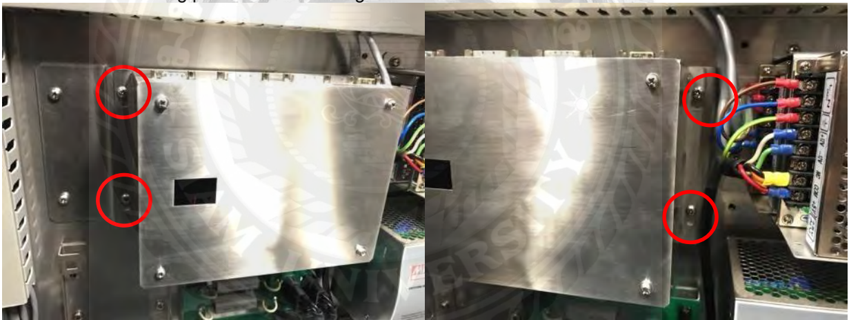
Figure 5-52 Location of Screws to be Tighten to Secure PLC to Bracket 1, PLC (E10-E14)
