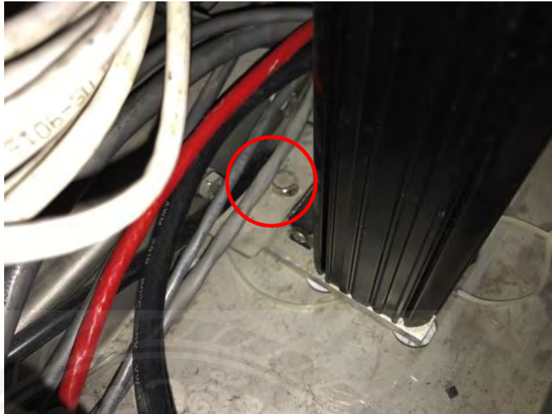
Figure 6-3 Location of the Bolt on the Stacker Clip
