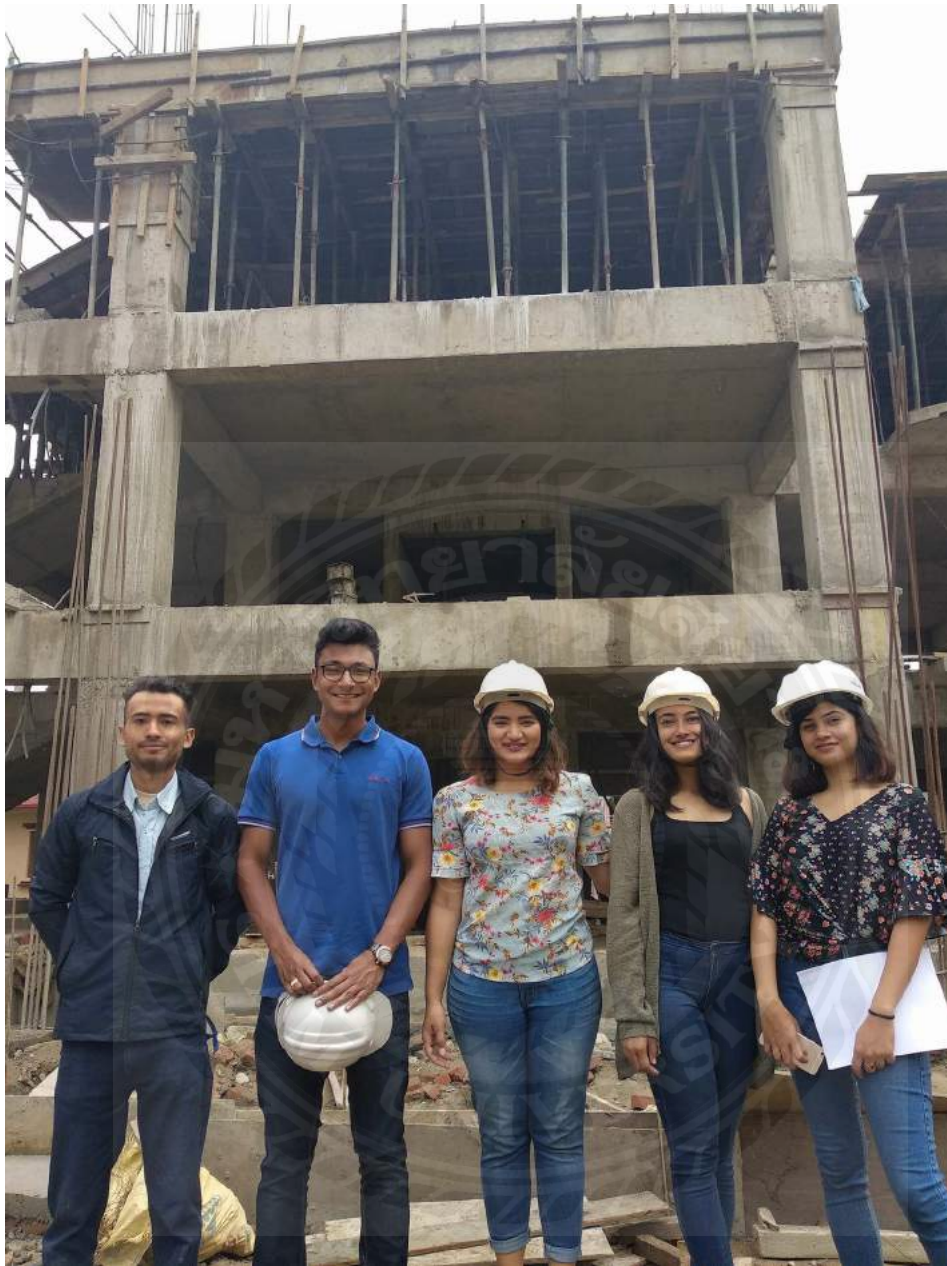
Figure 2: Construction site with the engineers
