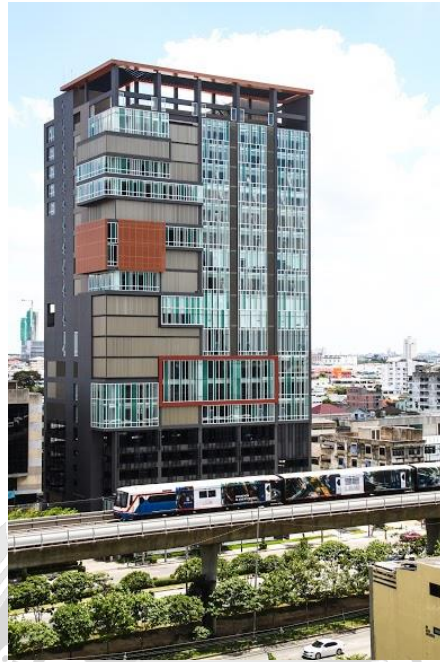
Figure 9. KX knowledge Exchange Building
