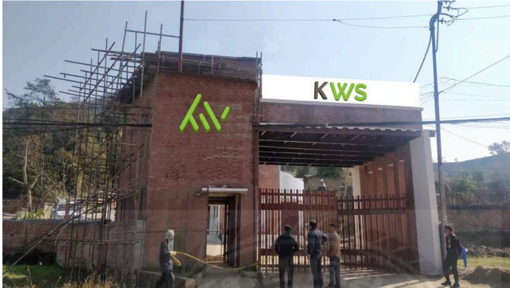
Picture 1.1 - Main Gate
