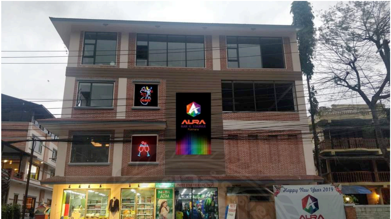
Picture 3.2 – Bars Exterior face
