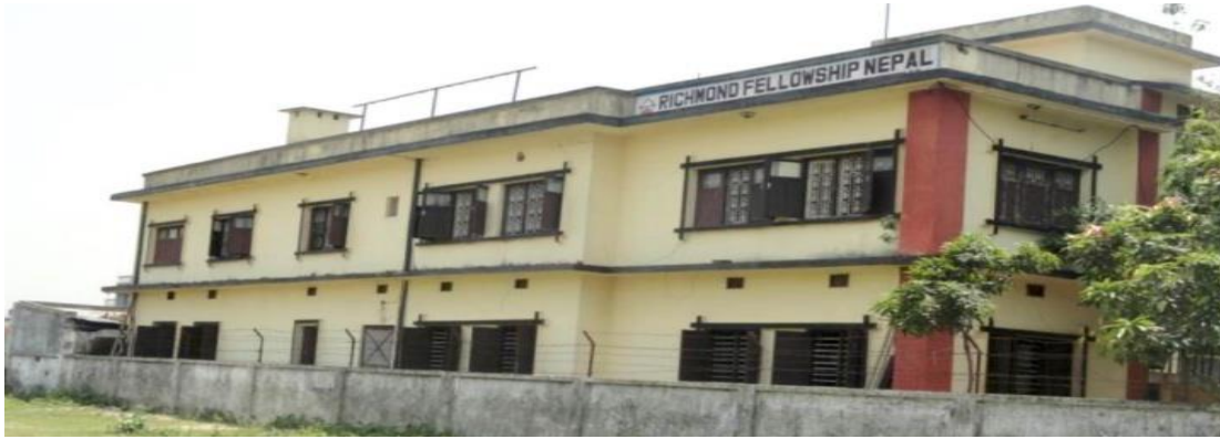
Annexure 1: Richmond Fellowship office where I worked for four months as an intern.
