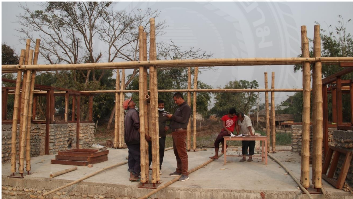
Figure 8: Photo taken during construction site work at madi, Hetauda
