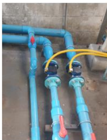
Ultrasonic water meter
