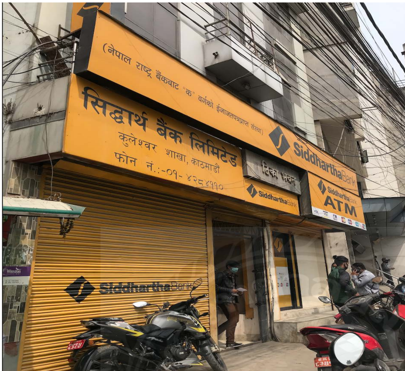
Figure 9: SBL branch at Kuleshwor, Kathmandu
