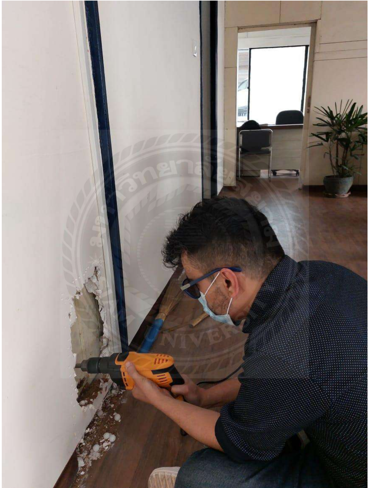
Image 10: Doing some maintenance work at the office in free time
