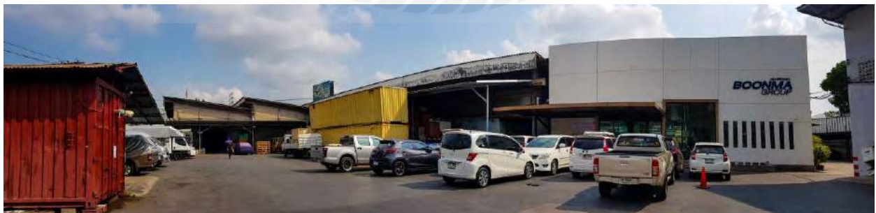
Figure 8: Company Building with Signboard
