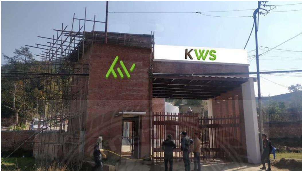
Picture 1.1 - Main Gate
