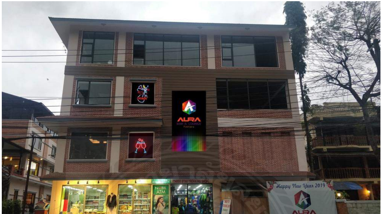
Picture 3.2 – Bars Exterior face
