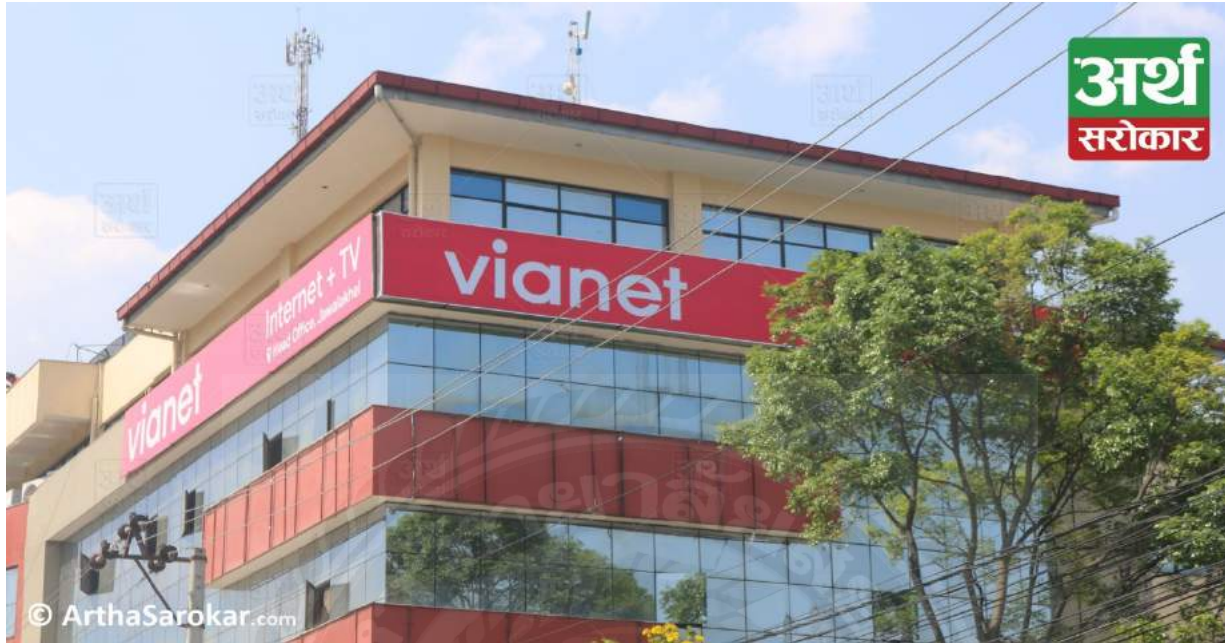
Picture 1: Vianet headquarter in Jawalakhel
