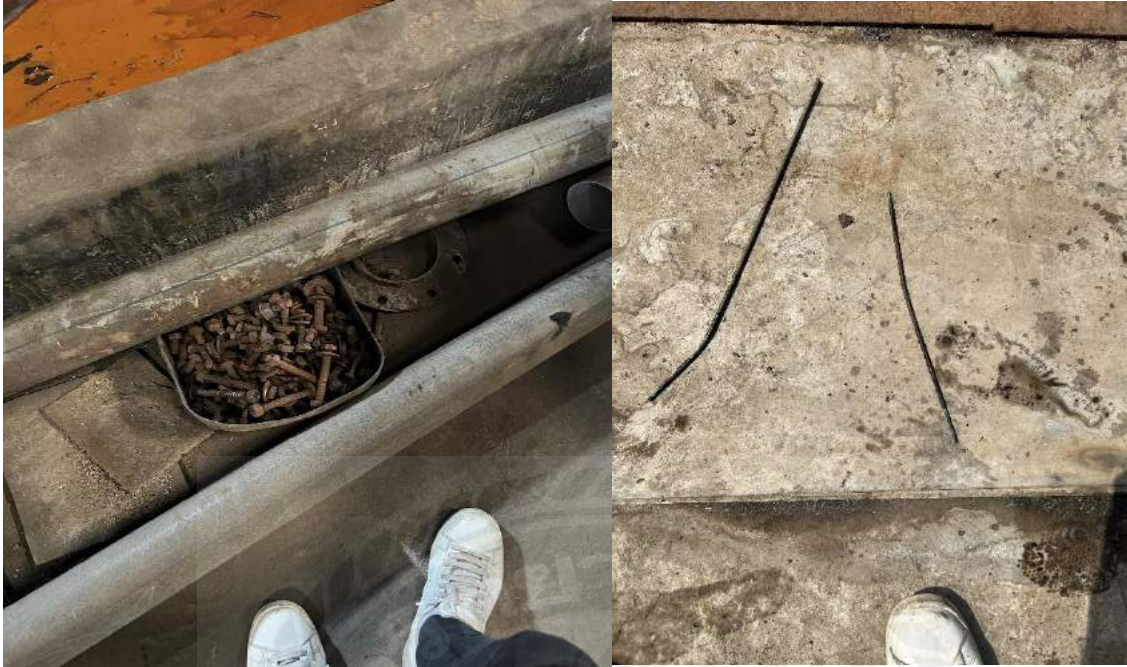
Figure 17: Wasted Nut bolt and welding rod.
