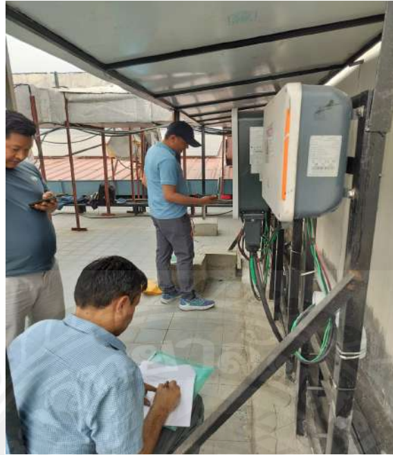
Figure 7: Monthly Inspection at the BBSM for the solar project
