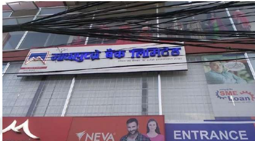
Figure 14 : Exterior view of Machhapuchchhre Bank Limited Kumariapati Branch
