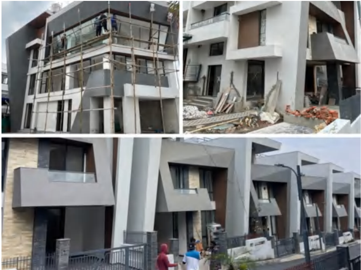
Figure 9: Pre- Handover Villa Inspection & Quality Assessment
